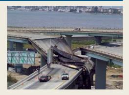
ration. Only one week after the accident, the lower I-880 connector had been repaired and was reopened. The I-580 overpass was completed in just 26 days, due in part to a bonus of \$200,000 paid for each day the work was completed sooner than two months after the accident. *Photo courtesy of California Department of Transportation, photographed by John Huseby*.
