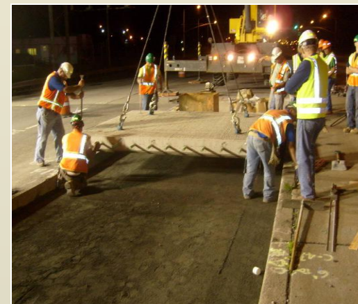
Replacing Existing Full Depth Asphalt
