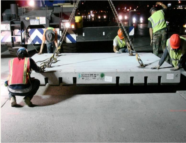
Center Slab in Hole (Single Slab Holes)
