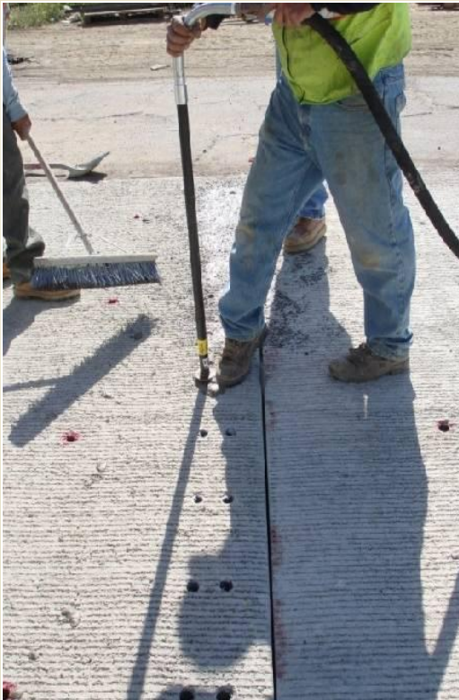
Fill Dowel Slots and Joints First
