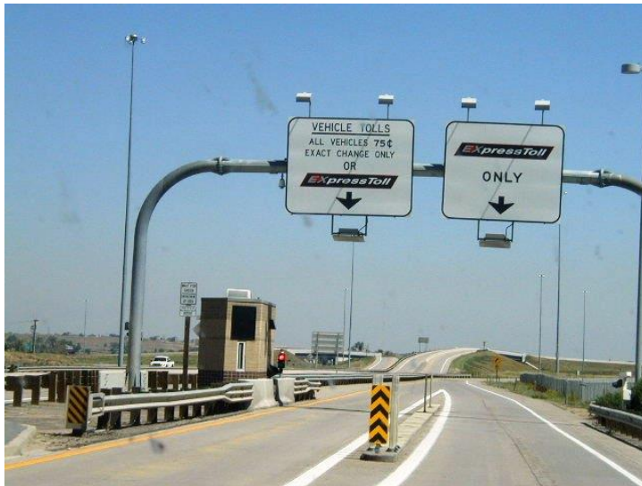
BEFORE – TYPICAL RAMP
