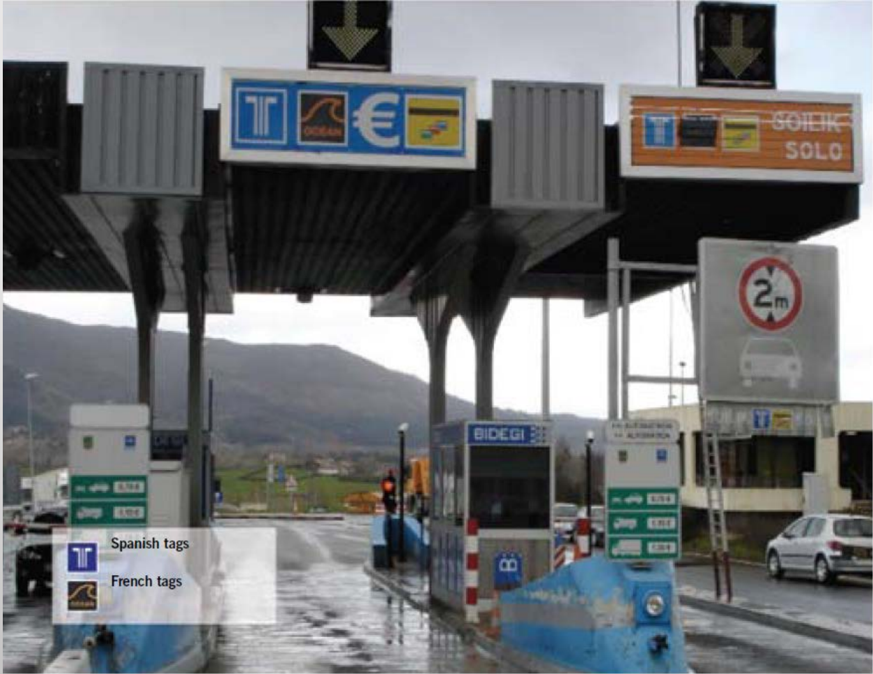
Irun Toll Plaza, A8, Spain
