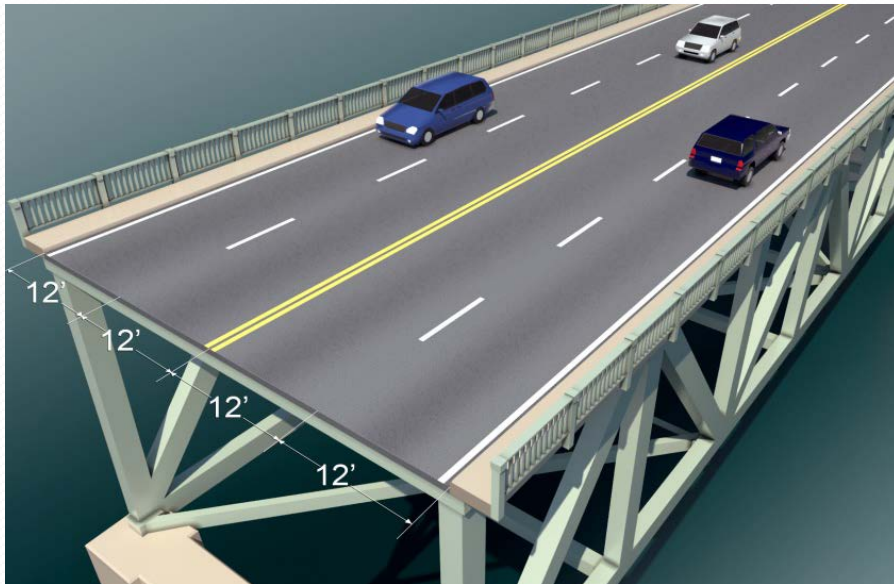
Existing lane widths
