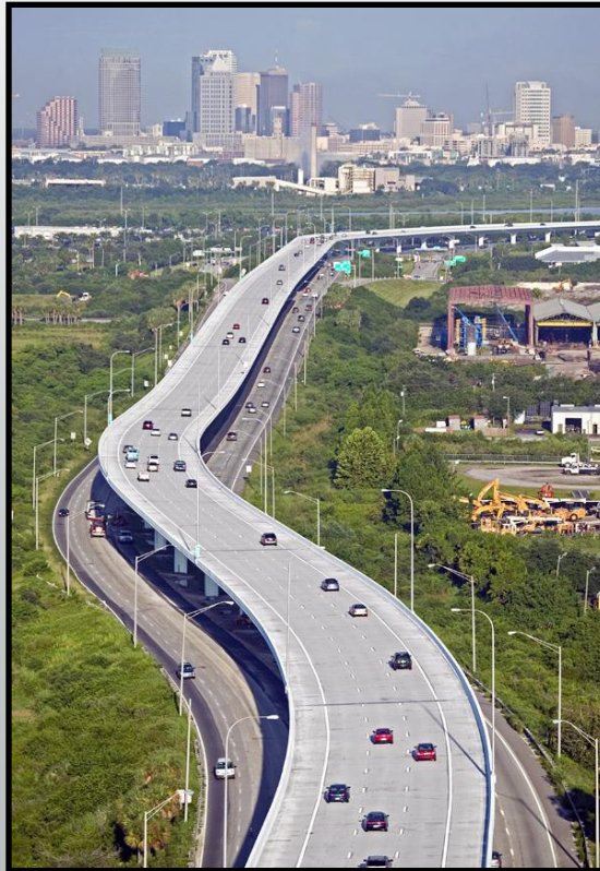
Tampa's Selmon Expressway Reversible Express Lanes
