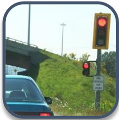
Adaptive Ramp Metering
