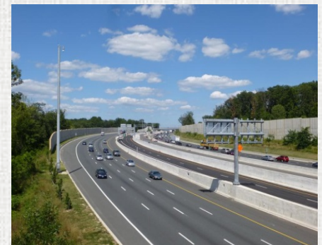
I-95 Express Toll Lanes (Completion 2014)
