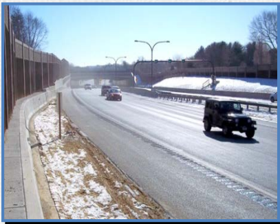
Intercounty Connector/MD 200 (Completion 2014)
