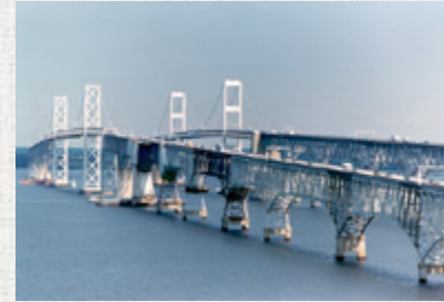
William Preston Lane, Jr Memorial Bridge (1952/1973)
