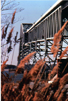
Harry W. Nice Memorial Bridge (1940)
