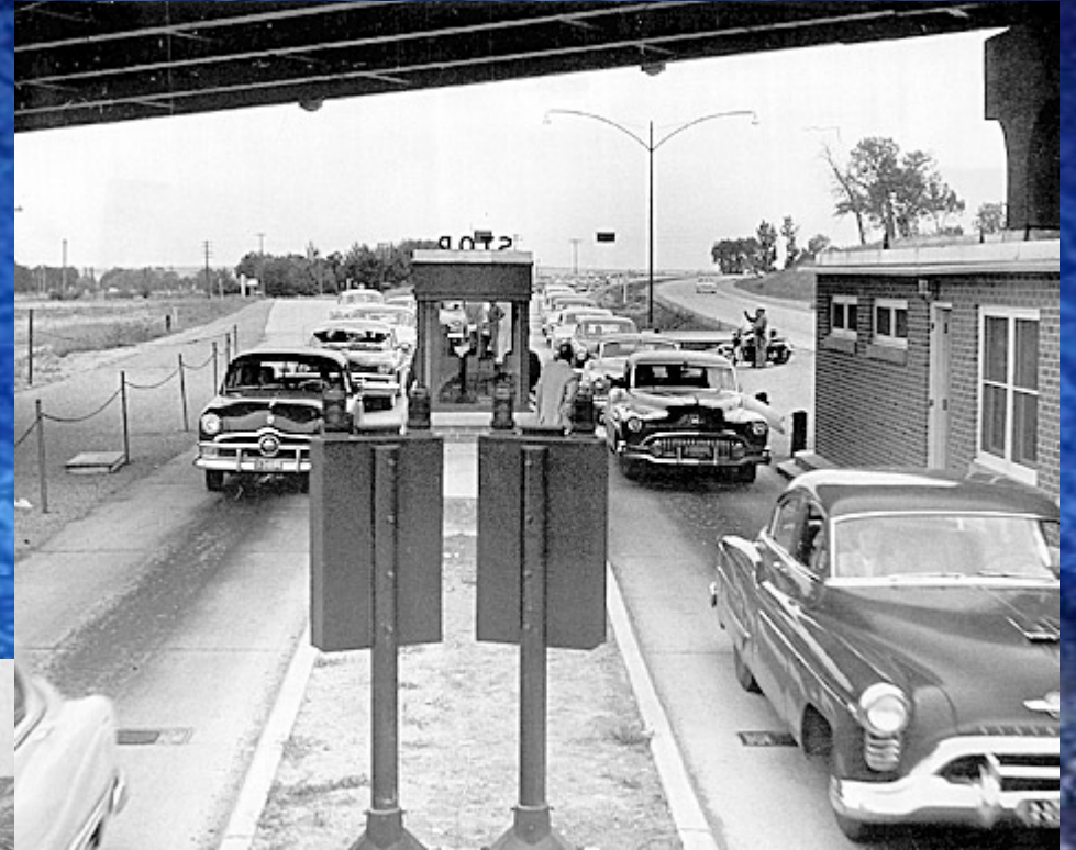
In 1953 the four-lane Denver-Boulder Turnpike lets you whiz over a former Indian trail.
