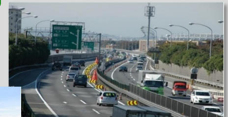
Lane Closure for maintenance works
