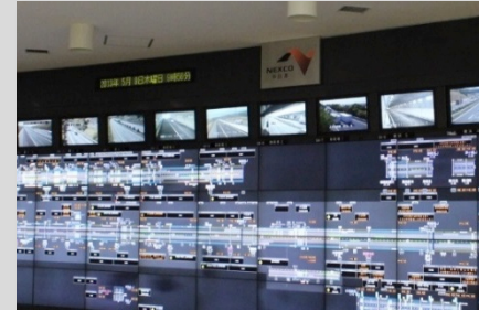
Traffic Control Center
