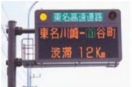
Variable Message Sign at IC Entrance
