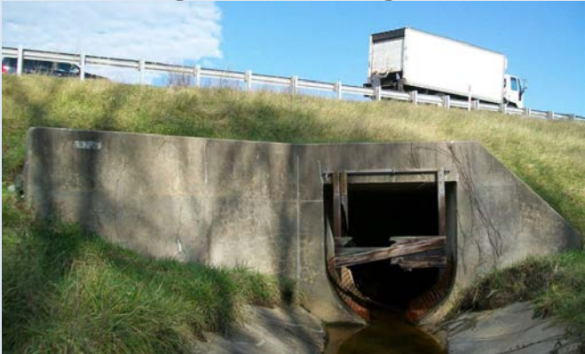
Small Bridges/Drainage (< 20 ft)
