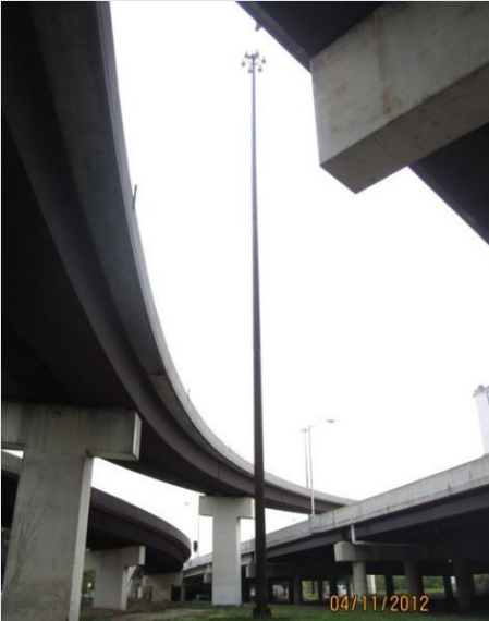
High Mast Light Poles
