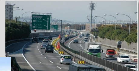
Lane Closure for maintenance works
