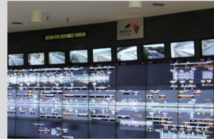
Traffic Control Center
