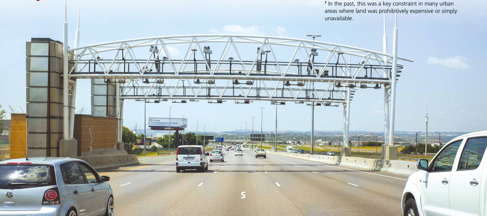
Figure 2: Freeflow Electronic Toll Collection
