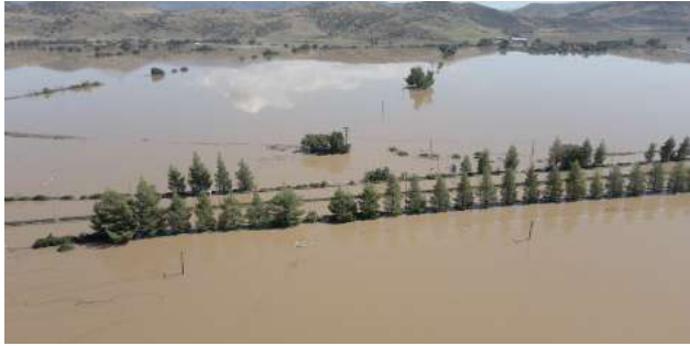
Area between Sykourio I/C – Gyrtani I/C: Flooded pavements
