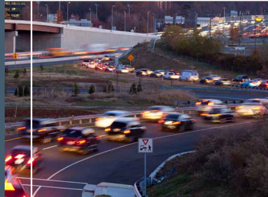
Capital Beltway/I-495 HOT Lanes, Fairfax County
