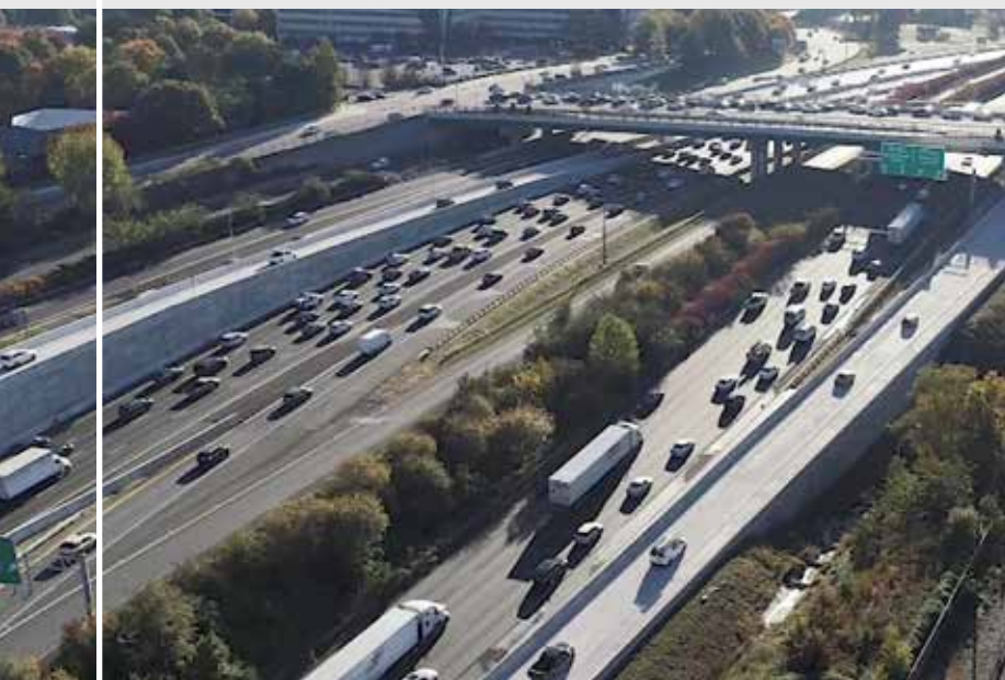
Northwest Corridor Express Lanes, Atlanta
