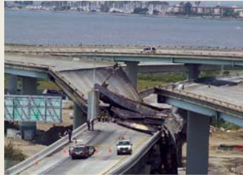
ration. Only one week after the accident, the lower I-880 connector had been repaired and was reopened. The I-580 overpass was completed in just 26 days, due in part to a bonus of \$200,000 paid for each day the work was completed sooner than two months after the accident. *Photo courtesy of California Department of Transportation, photographed by John Huseby.*
